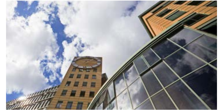
Solna Gate, the Aprikosen 2 property in Stockholm, is certified according to BREEAM In-Use Very good.
