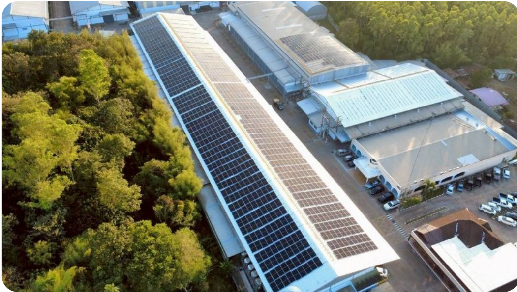
Solar panels on the roofs of our Prachinburi plant (Thailand.)
