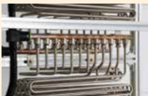
Liquid cooling device for data centers
