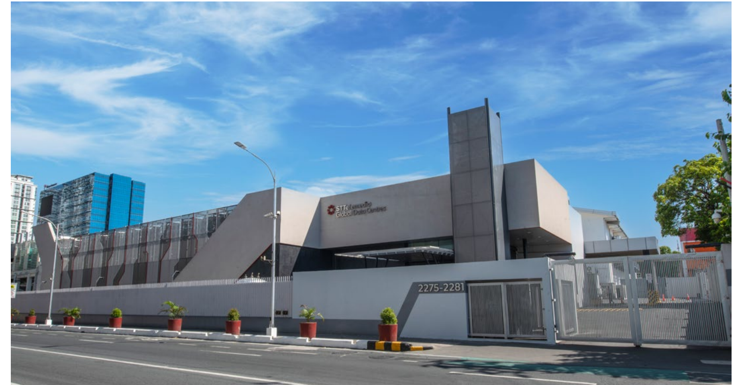
A data center of ST Telemedia Global Data Centres (STT GDC) in Makati, Philippines.
