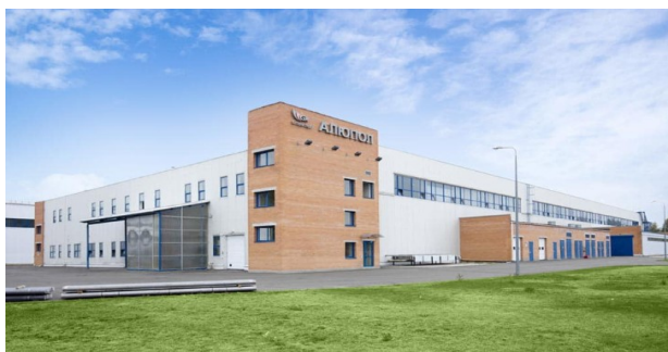
Plant in Borodianka
