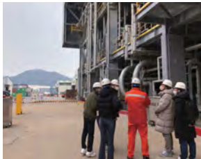
| On-site safety inspections
