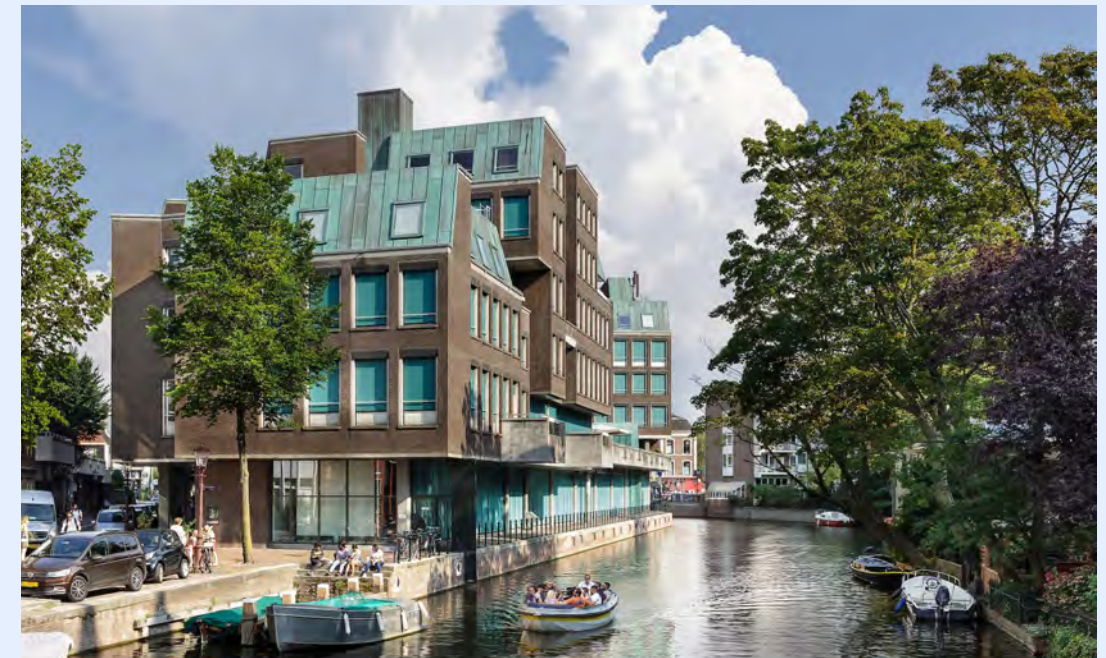
HECF piloted the draft C Change guidelines for transition risk at Noortse Bosch, integrating costs associated with decarbonization improvements into underwriting for the asset.
