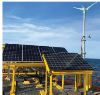
Wind Turbine Solar Hybrid Installation at SFJT-F (2 units).
