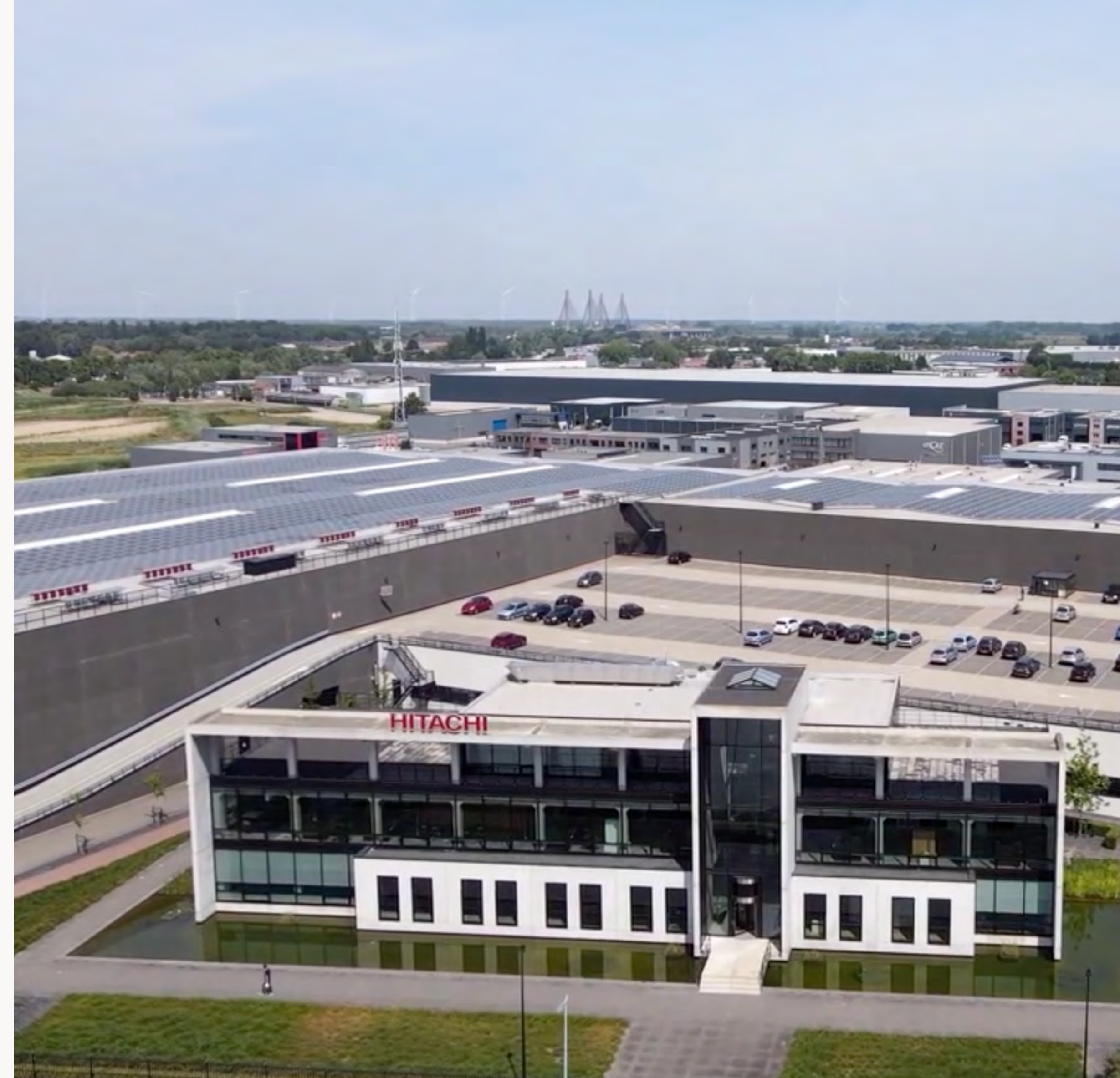
Hitachi Vantara's European Distribution Center in the Netherlands.
