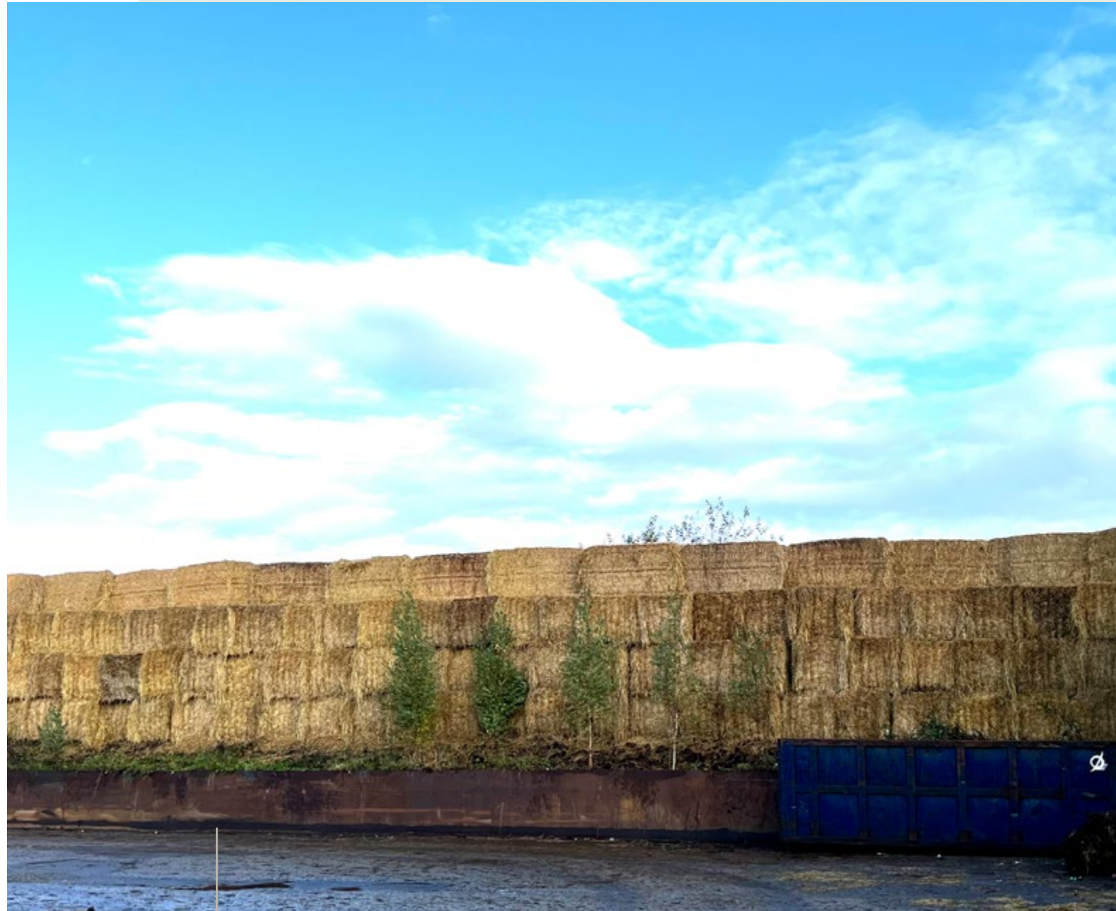
Image: The new straw bale noise barrier at the Odense site.
