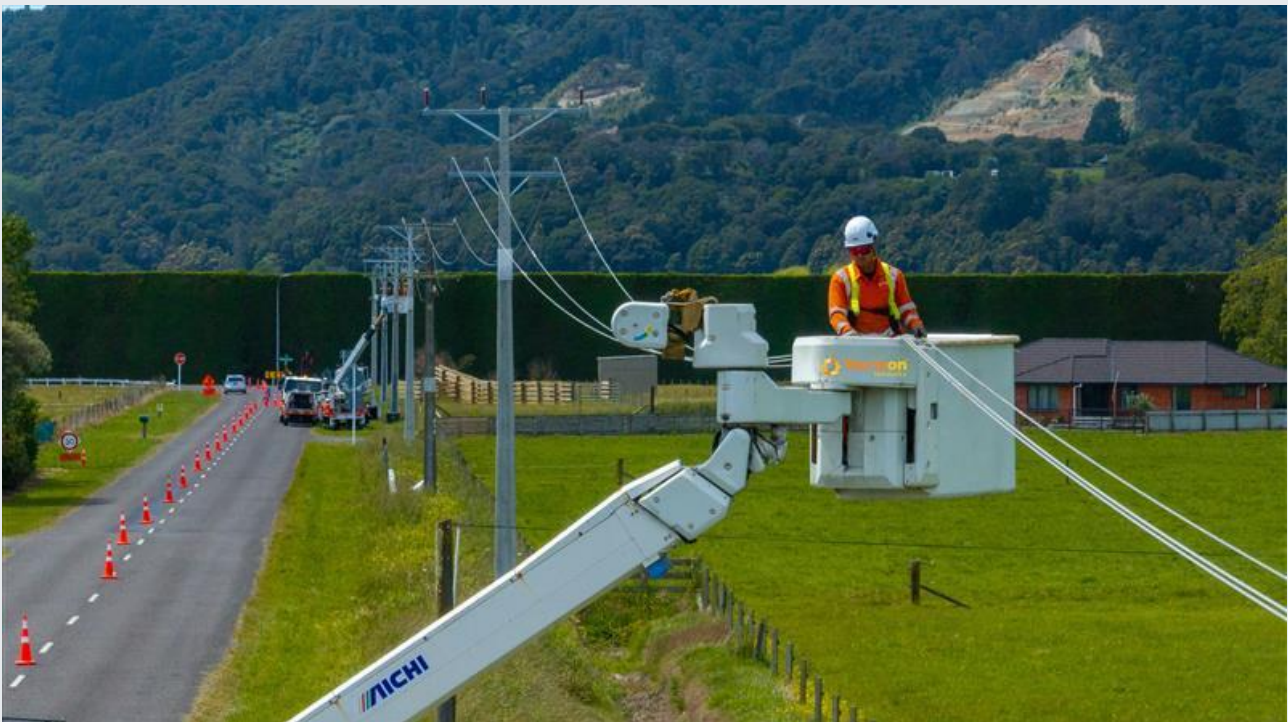
Picture: Safer Connections. Horizon Services at work, elevating infrastructure and safety in Whakatāne
