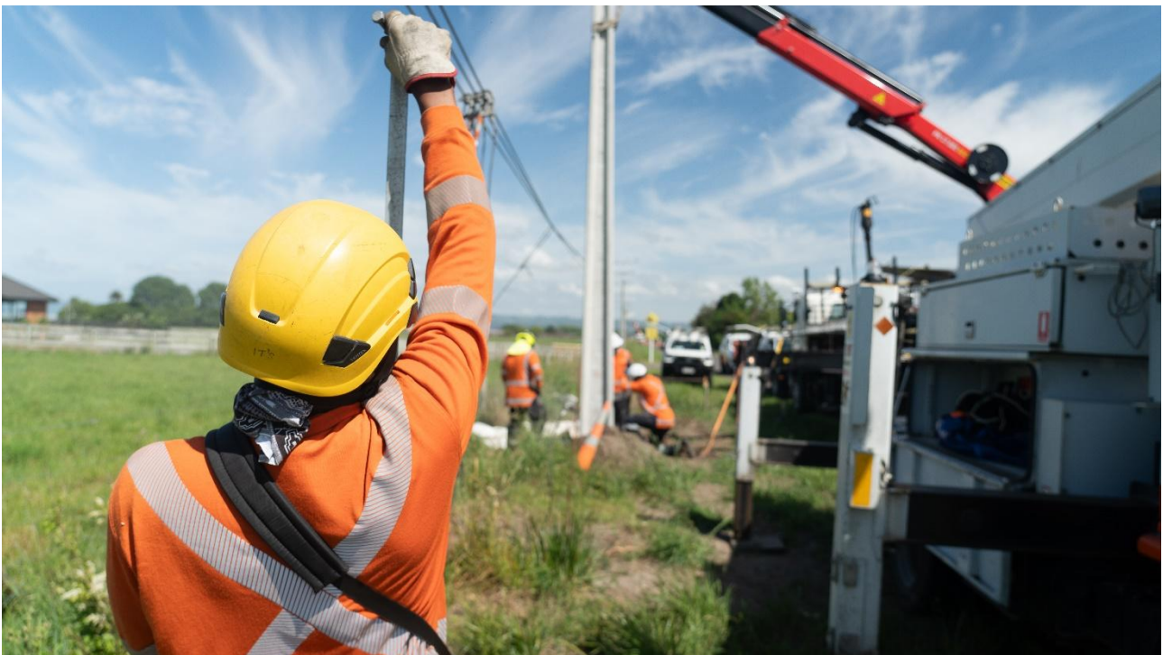
Picture: Horizon Services staff installing a pole.
