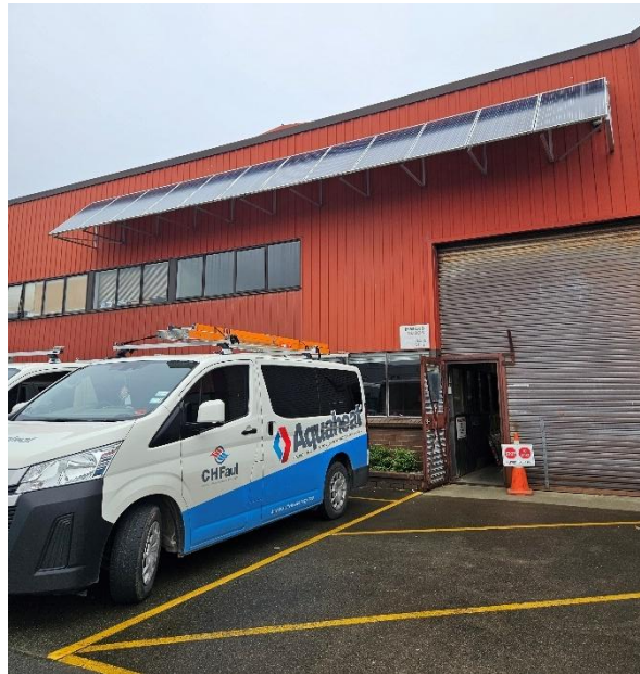
Picture: Solar panels for internal use of our Aquaheat's branch in Invercargill.
