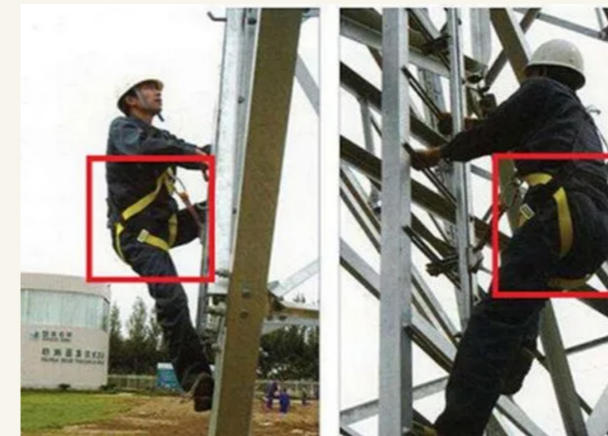
Delivery: An AI-based video system automatically checks whether workers are wearing personal protective equipment (PPE), making AI-assisted operations a reality.
