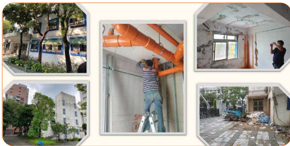
▲ Renovation of Wenshan Service Location
