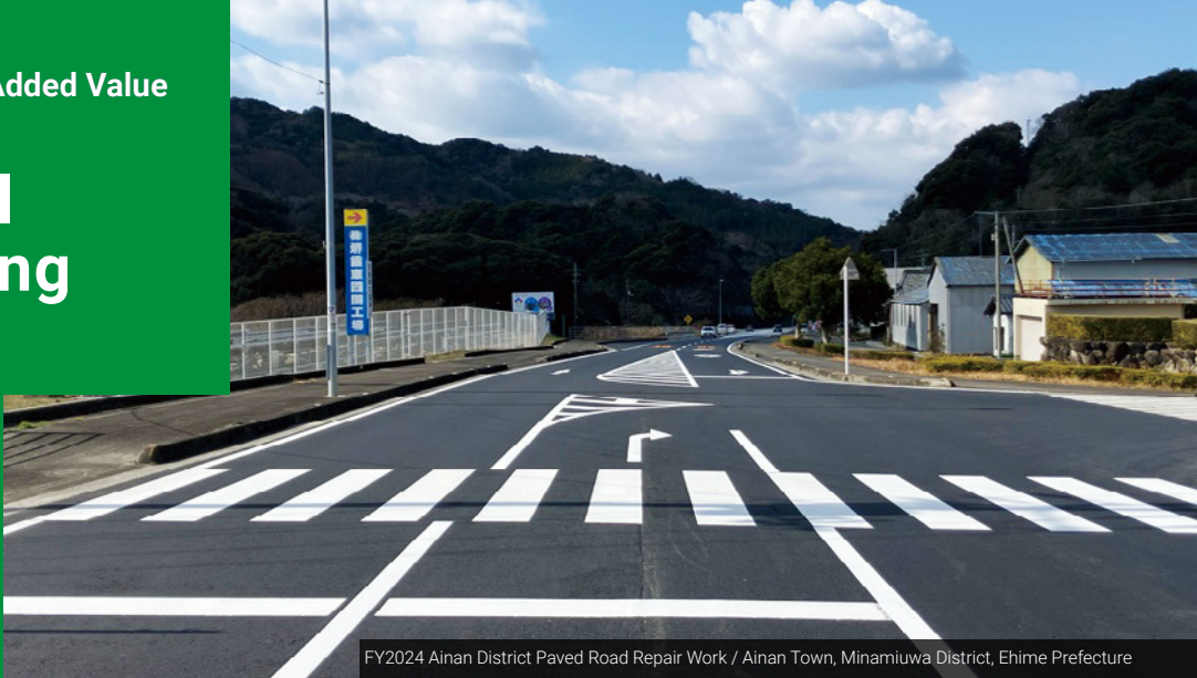
FY2024 Ainan District Paved Road Repair Work / Ainan Town, Minamiuwa District, Ehime Prefecture
