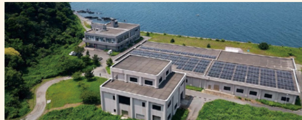
Miura City Public Sewerage (for East Area Treatment District) Management Business (management commenced April 2023 by a consortium including our Group)
