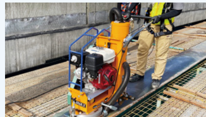
*3 Joint technical development with cooperating companies for H-beam surface cutting under bridge decks
