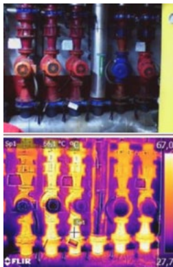
Before the insulation intervention
