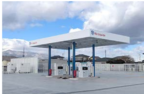
Motomiya Interchange Hydrogen Station
