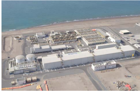
Aerial view of Oman seawater desalination plant
