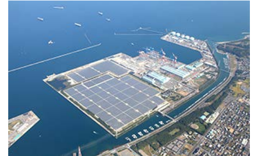
Oita-Hiyoshibaru solar power plant
