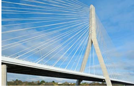
Structure made with blast furnace slag
