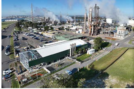
MCI's demonstration plant in Newcastle, Australia (photo taken in January 2025)
