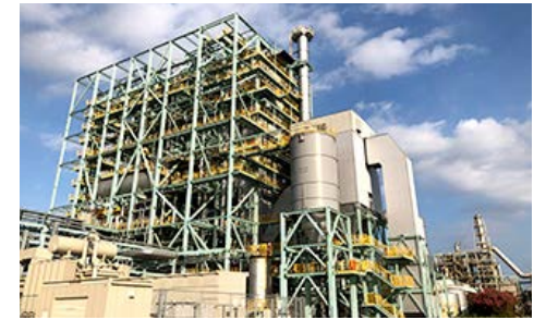
Exterior of Ichihara Biomass Power Plant
