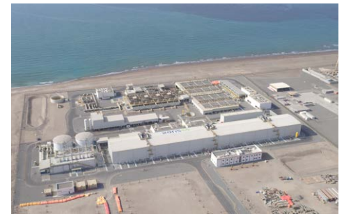
Aerial view of Oman seawater desalination plant
