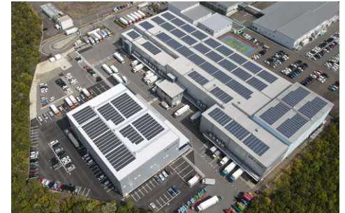
On-site distributed power supply operated by i GRID SOLUTIONS
