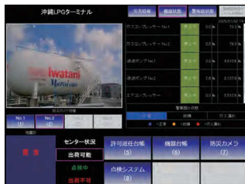
Centralized plant management using cameras
