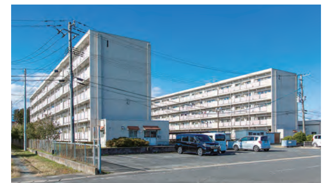
Homes in the city of Minamisoma participating in hydrogen-mixed LPG pipeline supply demonstration testing (80 units)
