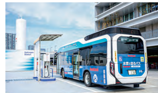
Iwatani Cosmo Hydrogen Station Ariake Bus Depot
