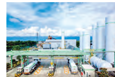
Industrial gas production plant
