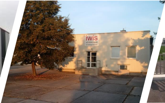
▪ Plant Strakonice, Czech Republic
