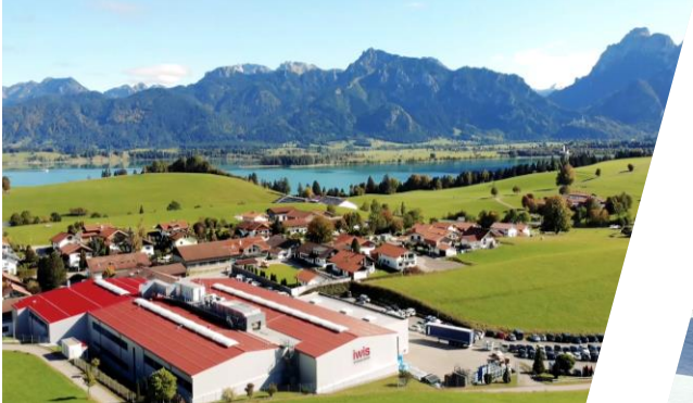
▪ Plant Rieden, Germany
