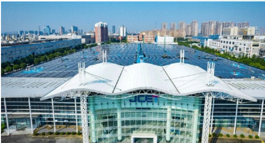
Official commissioning of JCET's 12 MW solar photovoltaic power station
