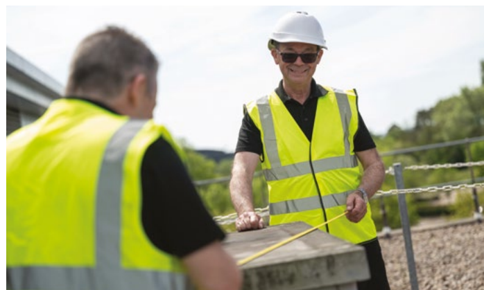
Investing in long-term sustainability: Colleagues measure up for our rooftop solar array at our Carlton Park Support Centre in the UK, which will support our clean energy goals.
