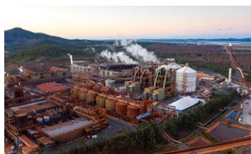
Planned construction site of alumina refinery plant
