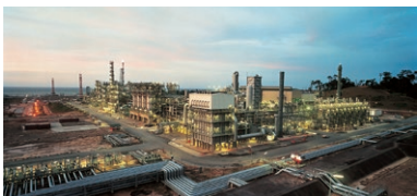
Large commercial GTL project in Malaysia
