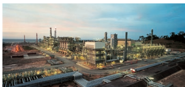
Large commercial GTL project in Malaysia
