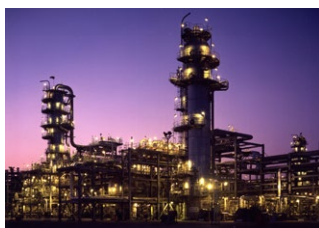
Gas processing plant (Saudi Arabia)
