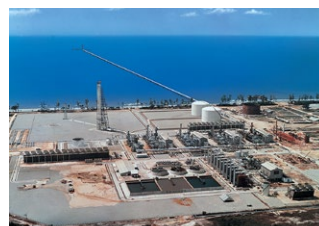
Our group's first LNG plant (Brunei)
