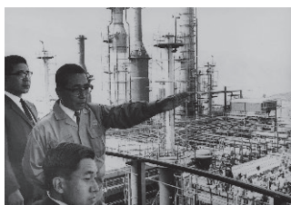
Refinery under construction (Peru)
