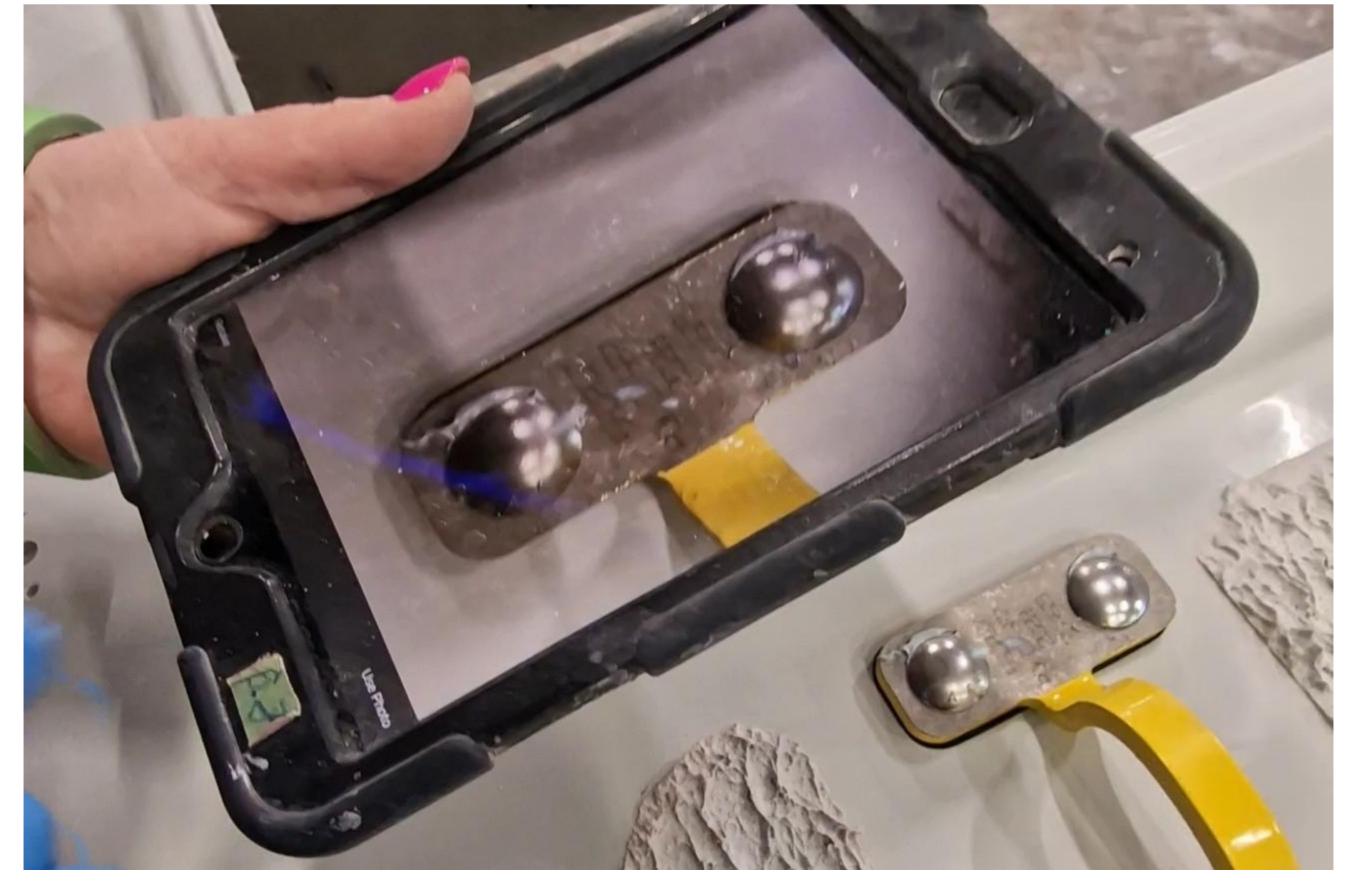
Anchor points inspection
