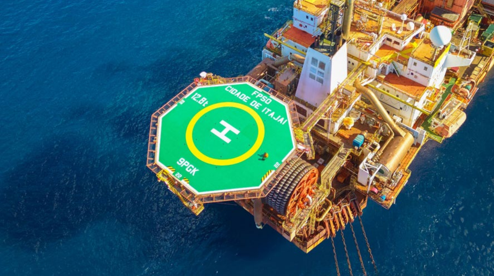
Baúna FPSO, Southern Santos Basin, Brazil
