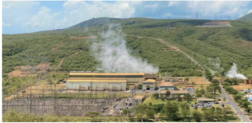
Olkaria II Power Station
