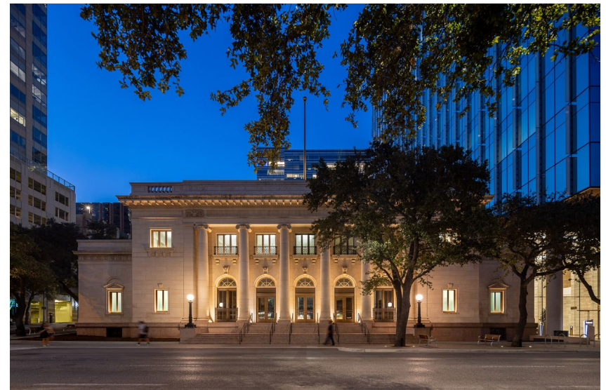
The Post, Austin, TX, Historical Preservation at Indeed Tower
