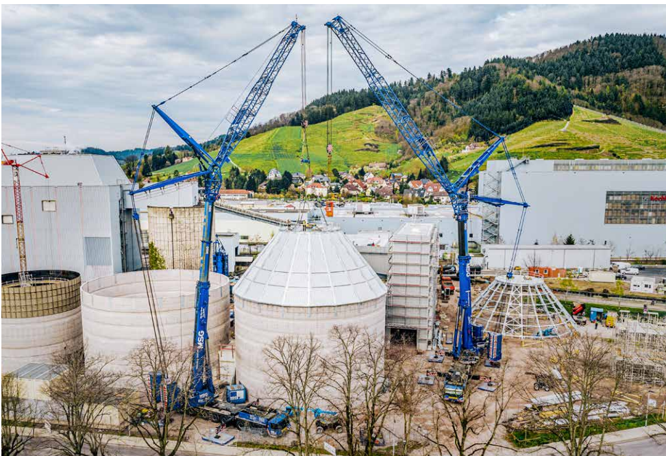
Four silos were built in order to store biomass.
