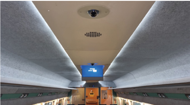
CCTV Installed in Cabin of KTX
