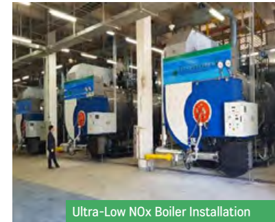
Ultra-Low NOx Boiler Installation
