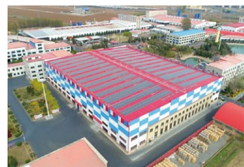
YKR's new No. 2 plant
