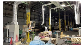
Installing air conditioners in work areas to prevent heat stroke We are also creating a comfortable workplace by striving to improve the work environment.
