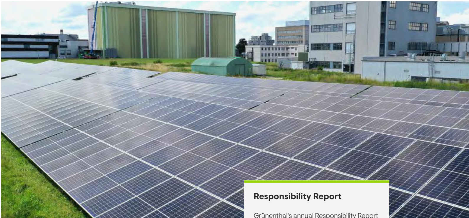
Solar power system at Grünenthal's headquarters in Aachen, Germany
