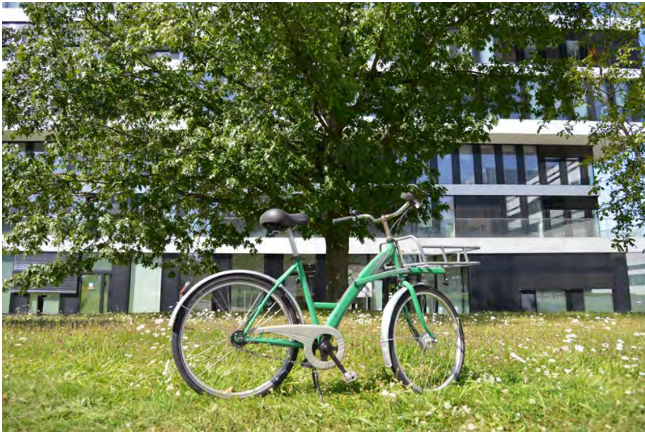
Aachen headquarters Campus
