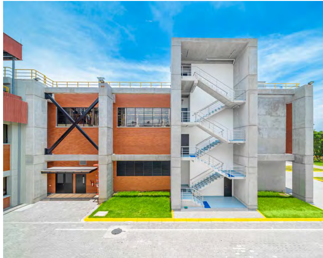
Built for excellence, designed for impact – the new plant at our Quito site
