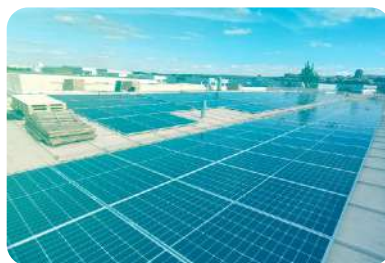
Toledo Plant Installation
