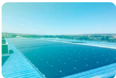
GRECO Warehouse Installation (Toledo)
