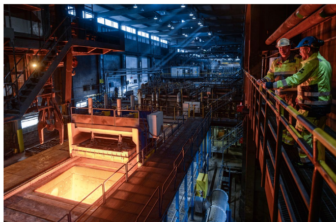
Linde's REBOX® oxyfuel reheating
