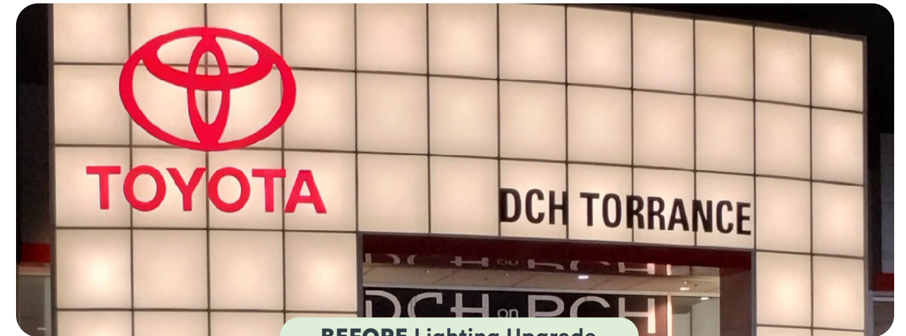
BEFORE Lighting Upgrade
