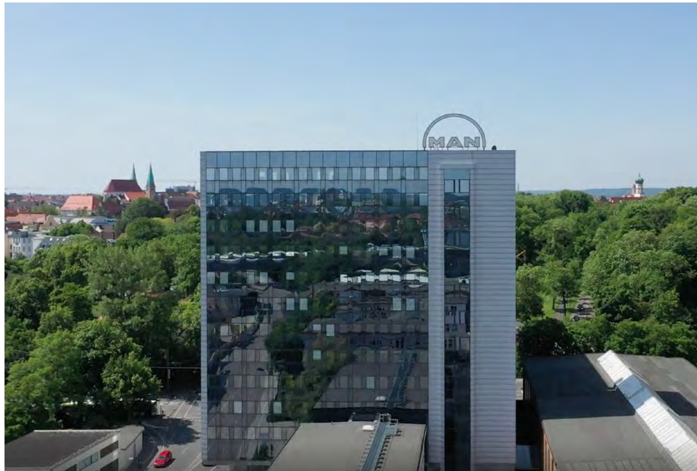
MAN Energy Solutions site Augsburg
