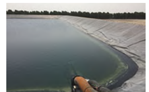
Lusail sewage treatment plant
