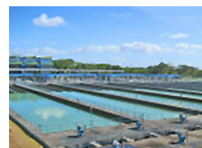
Maynilad Water purification plant
