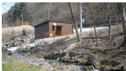
Small hydropower station (Hokuto City, Yamanashi Prefecture)
