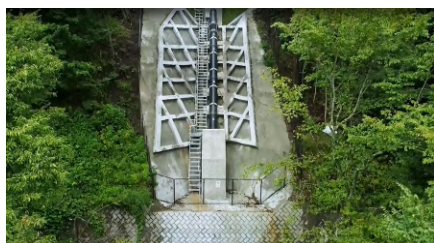
Tateshina Power Station No. 4 (Chino City, Nagano Prefecture)
