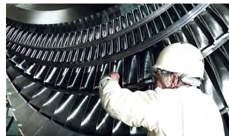
Turbine inspection in progress
