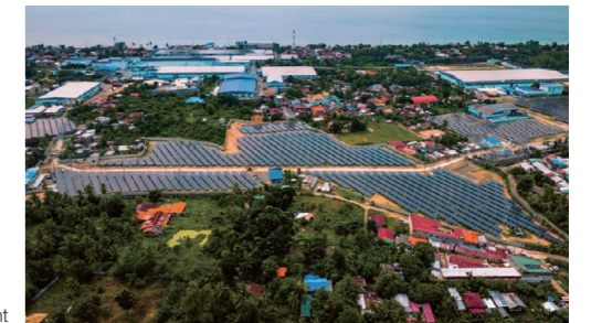
Solar power generation systems at the MITSUMI Cebu plant
