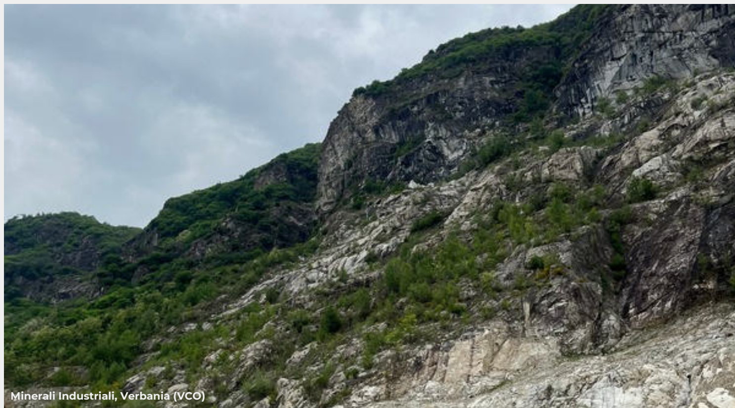
The site after our intervention
