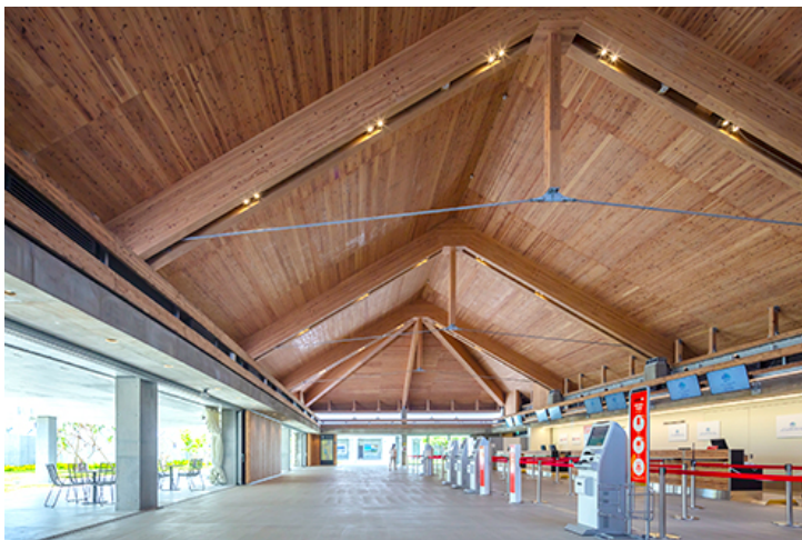
Miyako Shimojishima Airport Terminal
