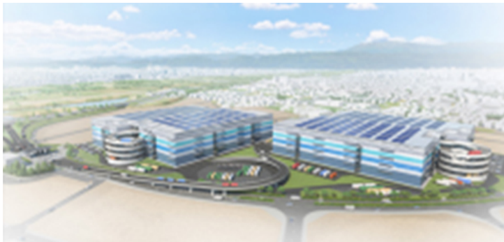
Image of a next-generation core logistics facility
