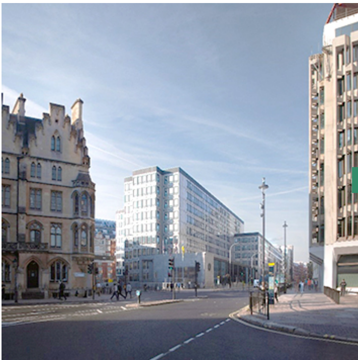
1 Victoria Street Original building
