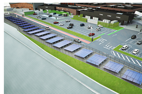
Installed solar panels (Fukaya-Hanazono Premium Outlets)
