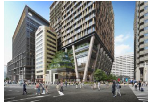
CLT panels and extensive green spaces on the lower floors of the building
