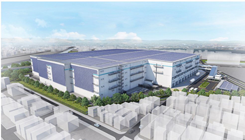
Solar generating equipment installed on the roof and walls of the building (conceptual rendering)
