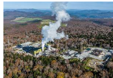
Appi Geothermal Power Plant (Iwate prefecture) Main business operator: Appi Geothermal Energy Corporation Operations scheduled to March 2024 Output: 14,900kW
