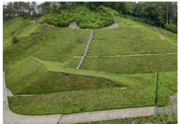
Contamination containment work (Komagi Mine) (Top: before work, Bottom: after work)
