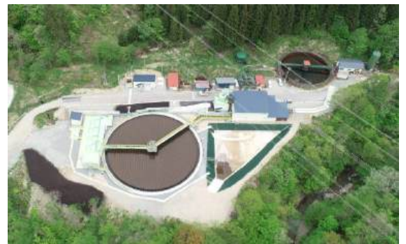
Acid mine drainage treatment facilities (Yatani Mine)
