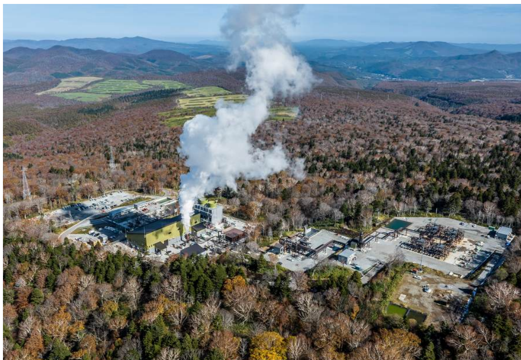
Appi Geothermal Power Plant
