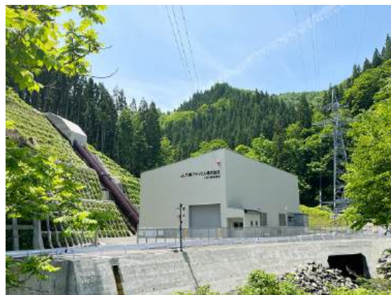
Komatagawa New Power Plant (Akita prefecture) Main business operator: Mitsubishi Materials Corporation Operation commenced in December 2022 Output: 10,326kW
