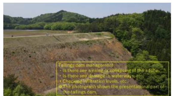
Example of tailings dam management (Osarizawa Mine)
