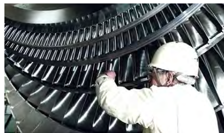
Turbine inspection in progress
