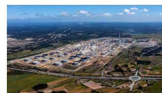
Galp's Sines refinery site for installation of new production facility
