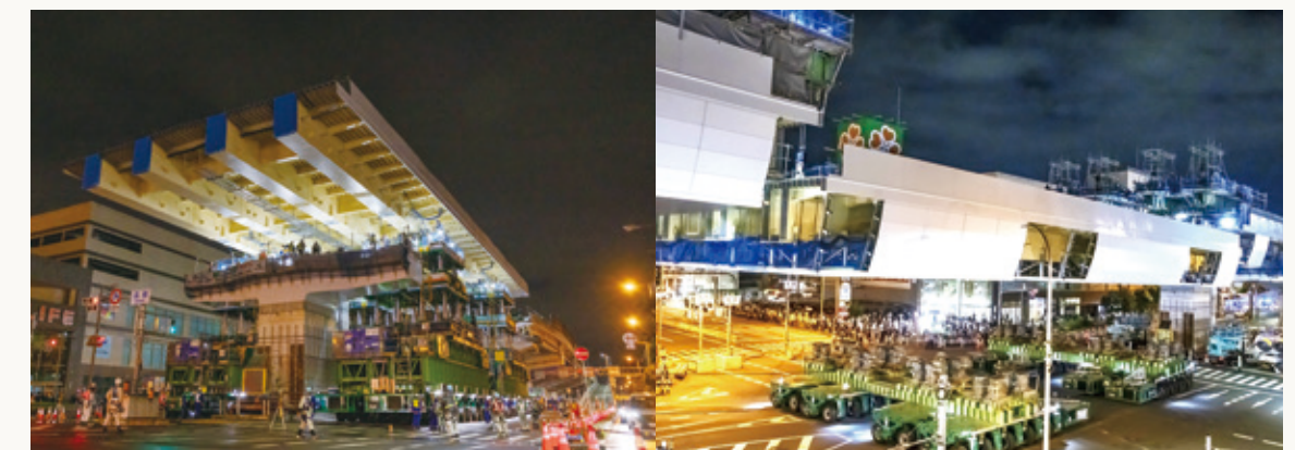
Launching erection of the bridge's side span
