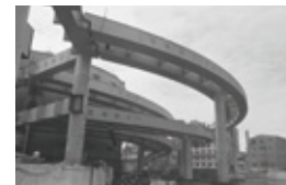
Edobashi Junction under erection work
