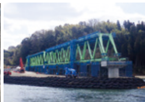
Progress with erection of the Kuma River Fourth Bridge (TT3/TT4)
