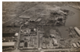
Suna-machi No. 1 and No. 2 Works
