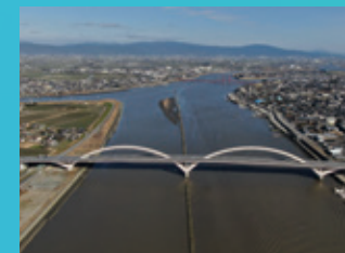
2021 Ariake Chikugo River Bridge
