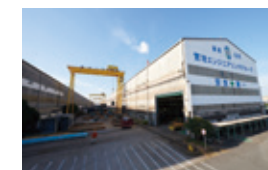
Chiba Works of MIYAJI ENGINEERING CO., LTD.
