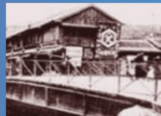
1868 Kurogane Bridge, Japan's first steel bridge
