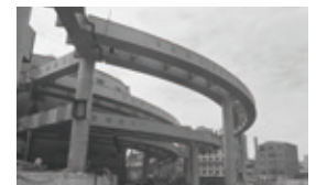
Edobashi Junction (under erection work)
