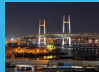
1989 Yokohama Bay Bridge
