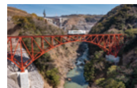
Minamiaso Railway's First Shirakawa Bridge
