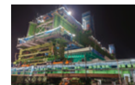
Chugoku Expressway Ishibashi Overpass Bridge (outbound line)
