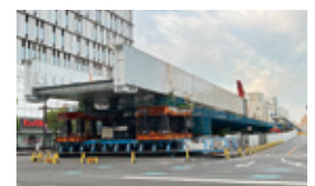
Elevation-related construction project at Hiroshima Electric Railway's Hiroshima Station
