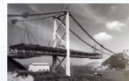
Kanmon Bridge under erection work
