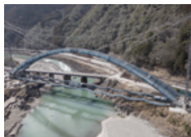
Progress with erection of the Kamase Bridge
