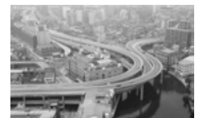
Edobashi Junction (completed)
