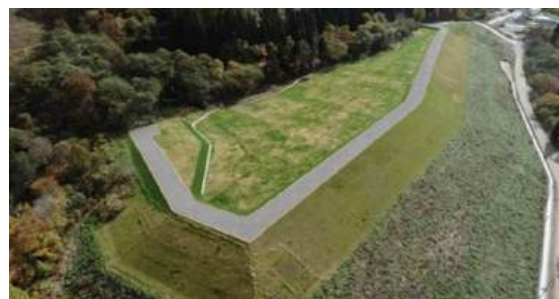
Reinforcement work by soil stabilization at the Yatani Mine Tailings Dam (completion)
