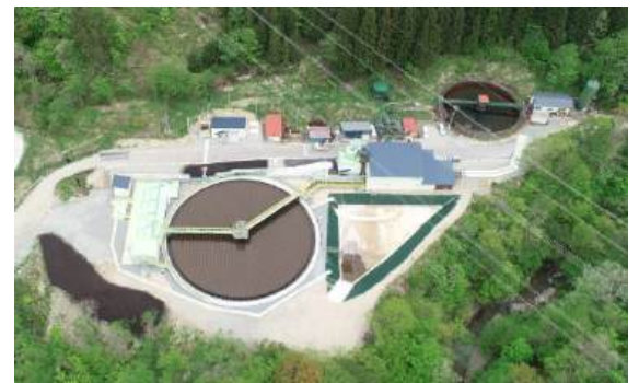
Acid mine drainage treatment facilities (Yatani Mine)
