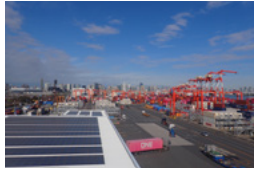
Solar power system at Tokyo International Container Terminal
