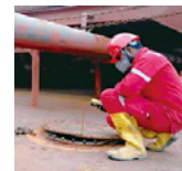
Gas detection in a tank before work
