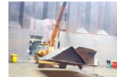
Dismantling operations in cargo hold
