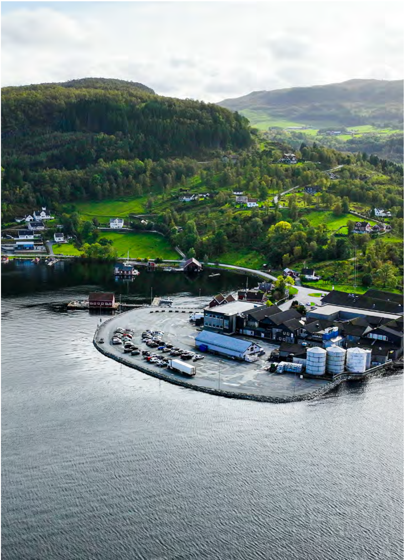
Ryfisk primary processing facility, Mowi Norway South
