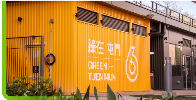
GREEN@TUEN MUN, re-provisioned by MTR, features sustainable design, including solar panels and sitting out area for residents
