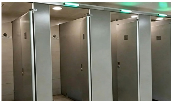
Smart restroom to show the real-time occupancy of the toilet
