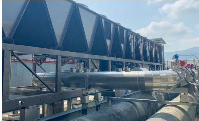
Chiller replacement at Kam Sheung Road Station
