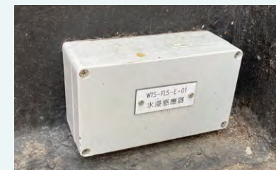
Installation of flooding sensors at station entrances or exits
