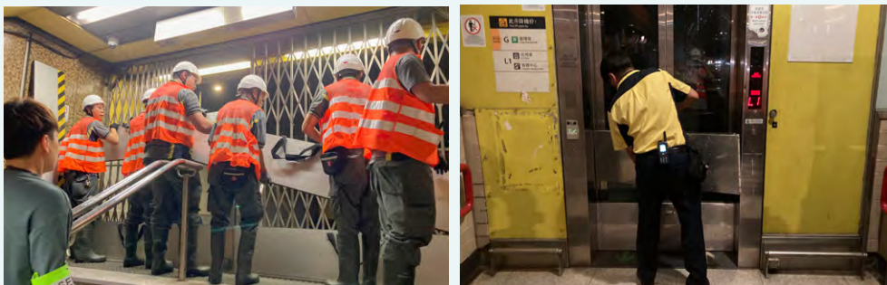
Installation of flood boards at Wong Tai Sin Station
