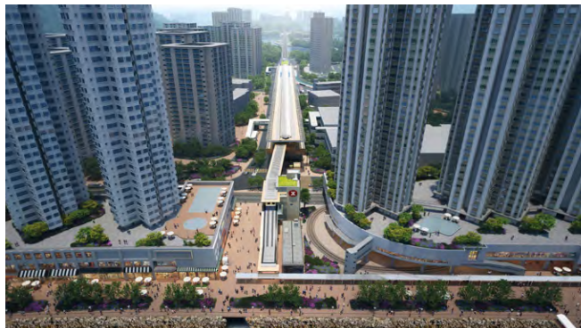
Artistic impression of the compact design of Tuen Mun South Station* to minimise the occupied road area and to make good use of natural ventilation corridor for natural airflow and convection for the station
